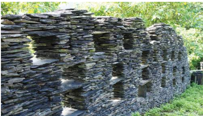
Sacrificial head wall
