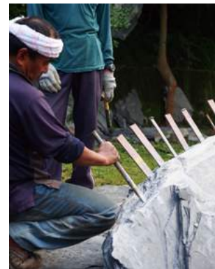
Building of a slate house
